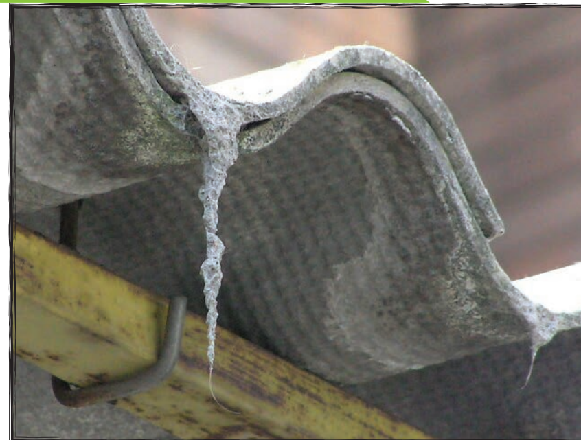
CHAPAS DE FIBROCEMENTO (ASBESTO-CEMENTO)
